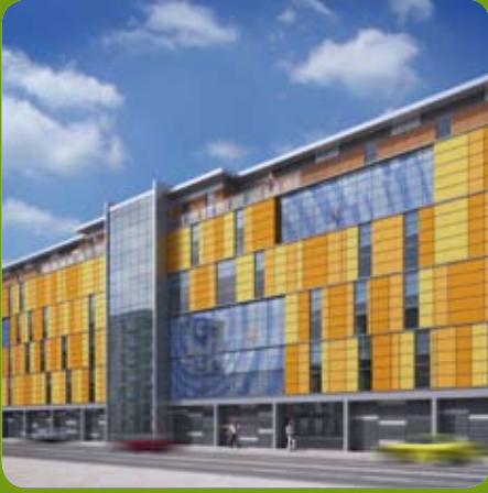
Above: Colston Primary Care Centre, currently in development
